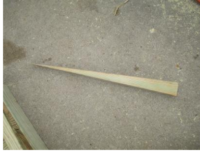
Figure A8. Cut 3 wedges for TA stringers.
