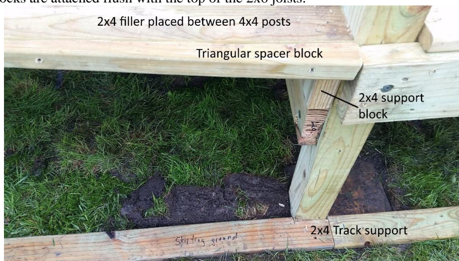
Figure D1. 2x4 filler, triangular spacer block and track support
