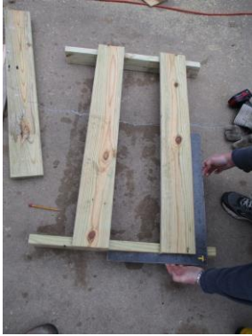
Figure A7. Screw deck boards to toe boards while upside down.
