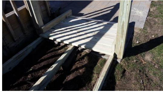
Figure 7. Stringers into Ramp end post assembly.
