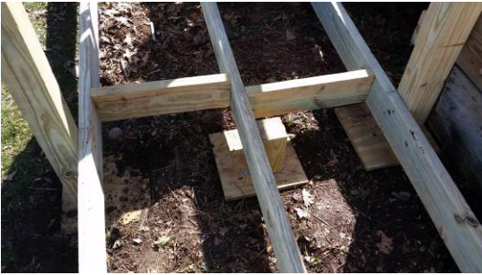
Figure 8. Ramp frame. Notice cross braces.
