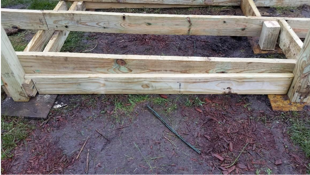
Figure D5. Vertical deck board fills a narrow gap at the end of the ramp instead of a skirting panel
