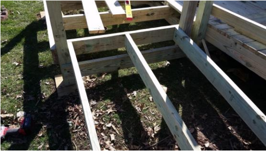
Figure 6. Ramp frame with 180° landing. Notice cross bracing
