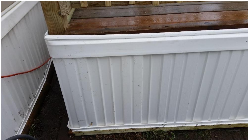
Figure D6. Completed skirting.
